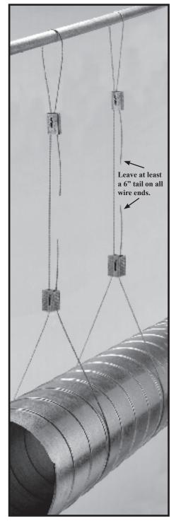
As a matter of sound engineering practice, the Rize Kwik-Loc assembly must be located no closer than 12 inches to the suspension point. In the case of round duct, where the wire rope encircles the duct, the Kwik-Loc must be located the distance of one diameter from the duct wall.
