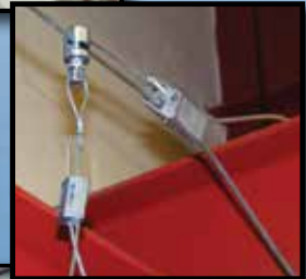
CAT LOC ON HORIZONTAL CABLE
